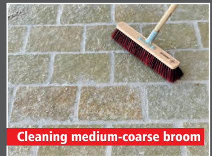
Filling the joints
